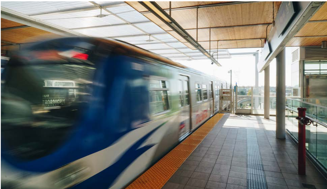
Figure 34: Marine Drive Canada Line station
