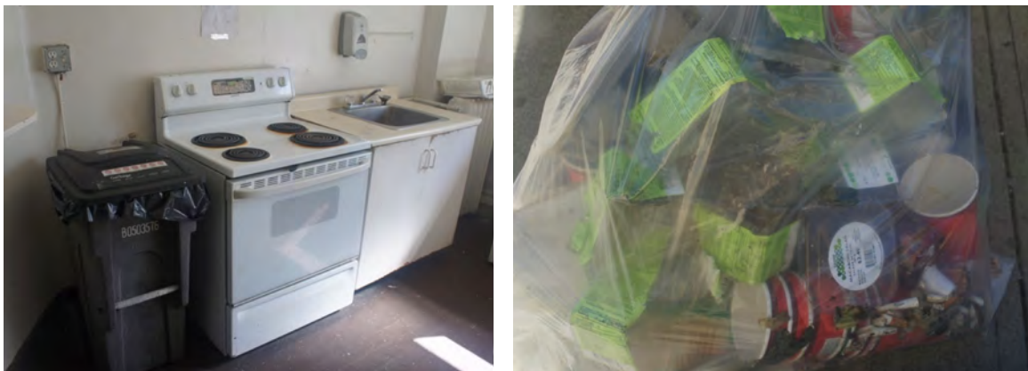
Images: A shared kitchen in an SRO lacks compost and recycling receptacles, and a garbage bag from another SRO is completely full of recyclables. When buildings have only single-stream waste service, residents have no option but to put everything in the garbage.
