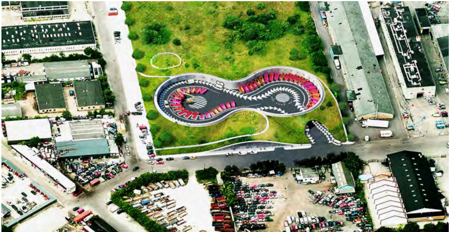
Image: Plans for a new residential transfer station in the urban neighbourhood of Sydhavn, Copenhagen (photo credit: Bjarke Ingels Group).
