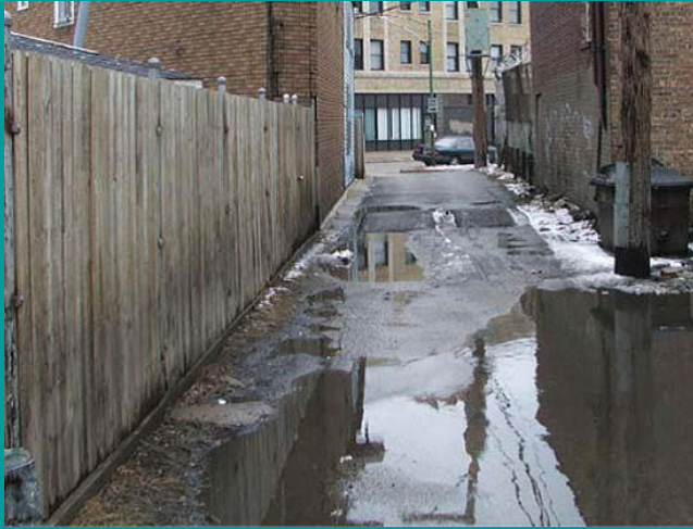
Alley with impermeable pavement and poor drainage Image from CDOT, 2010
