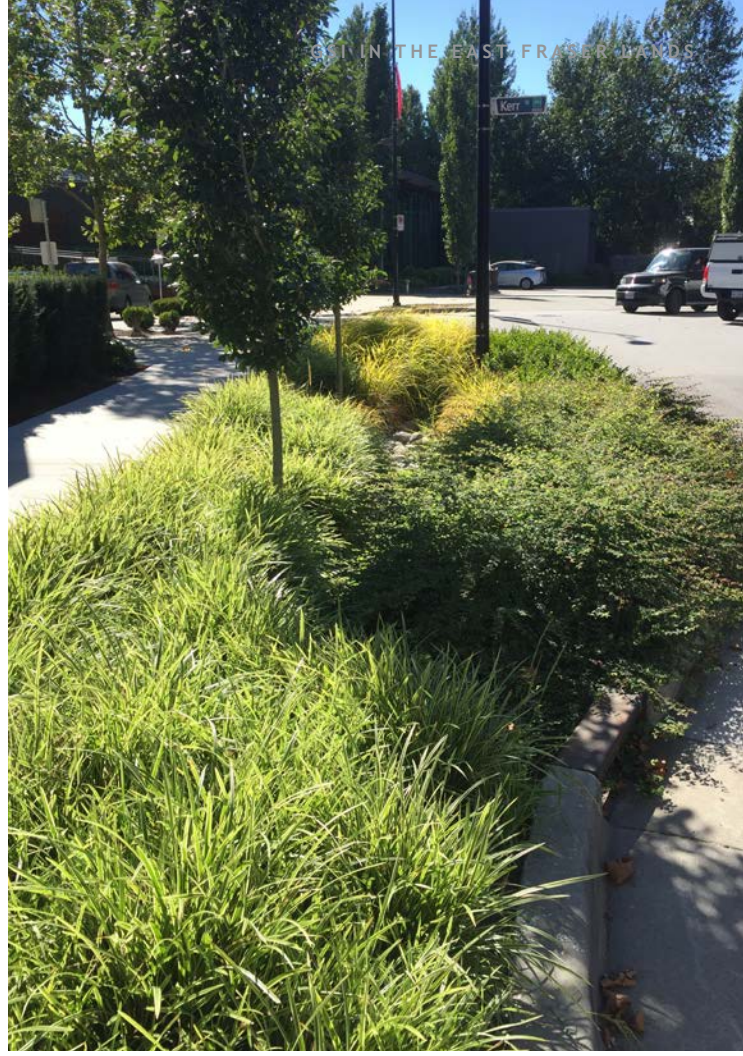
A rain garden in the EFL
