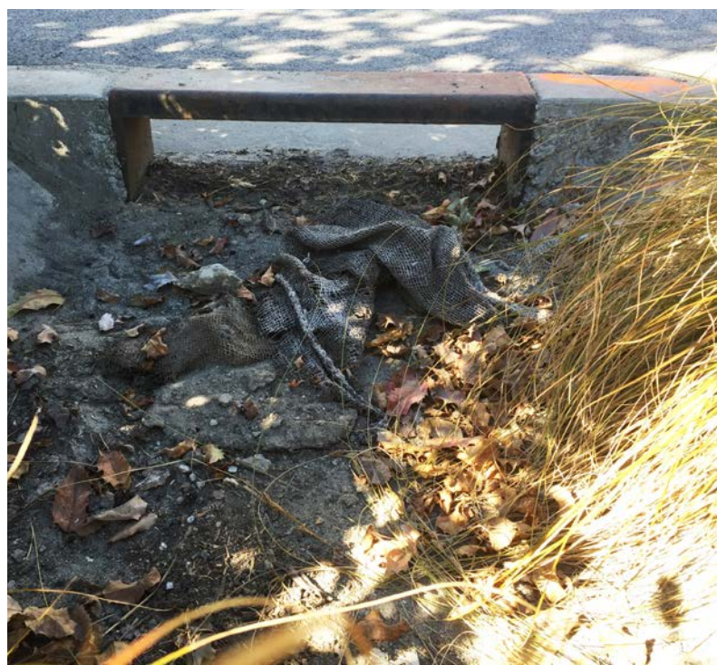
Rain gardens in the EFL getting clogged by sediment, leaves, and litter
