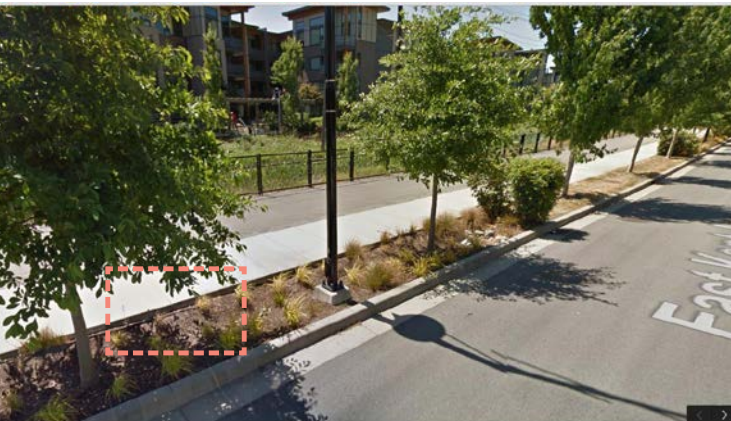
Grass boulevards with possible tripping risks
