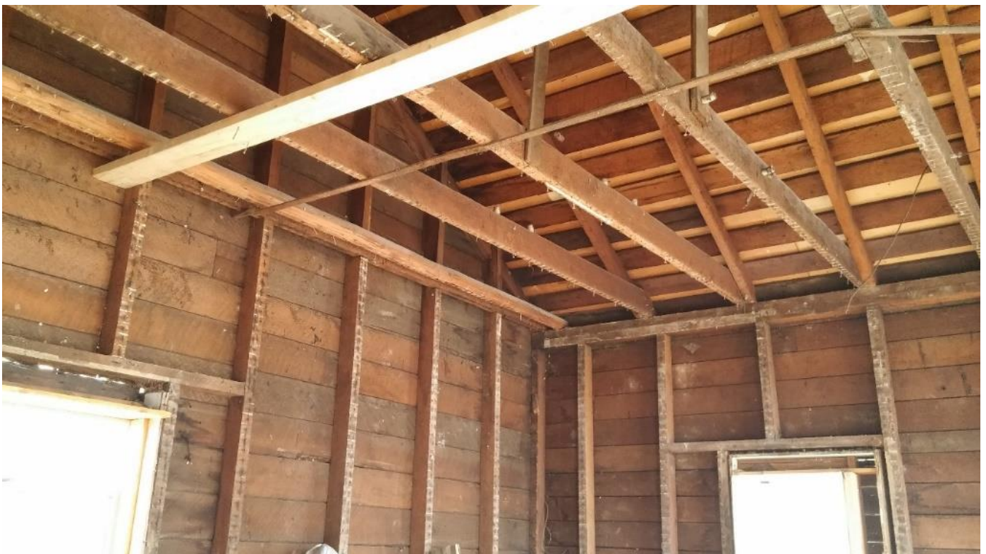
Figure 4 Framing structure (2×6 joists and rafters, 2×4 studs, and sheathing) of a 1920s house
