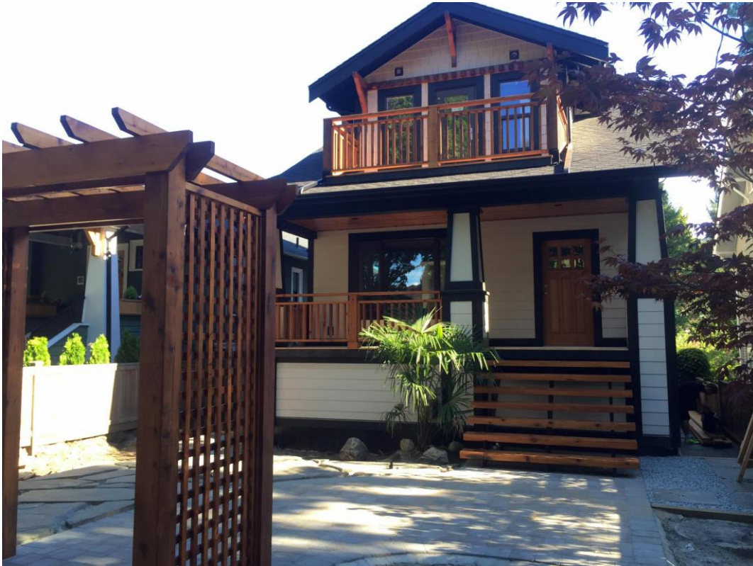
Figure 26 Exterior elements from salvaged wood ( Naturally Crafted Construction )
