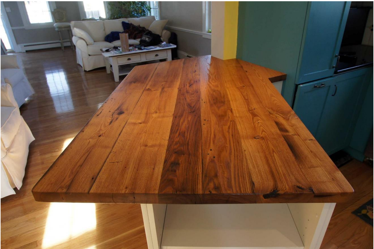
Figure 23 Countertop made from reclaimed wood (retrieved from the link )
