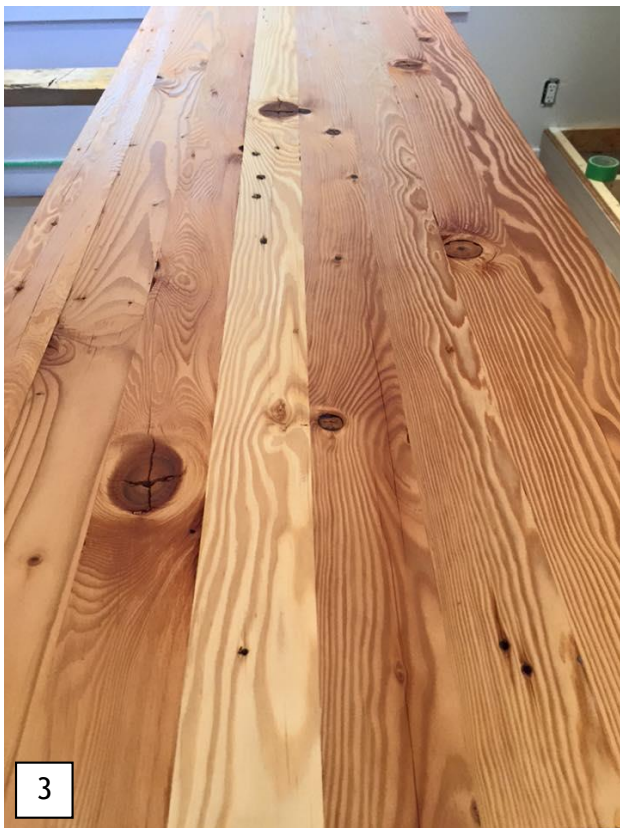
Figure 11 Planning, gluing, and refinishing of 2x4s to be reused as stair tread (by: Naturally Crafted Construction )
