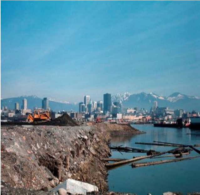
Fig. 55. Construction of the Seawall I
