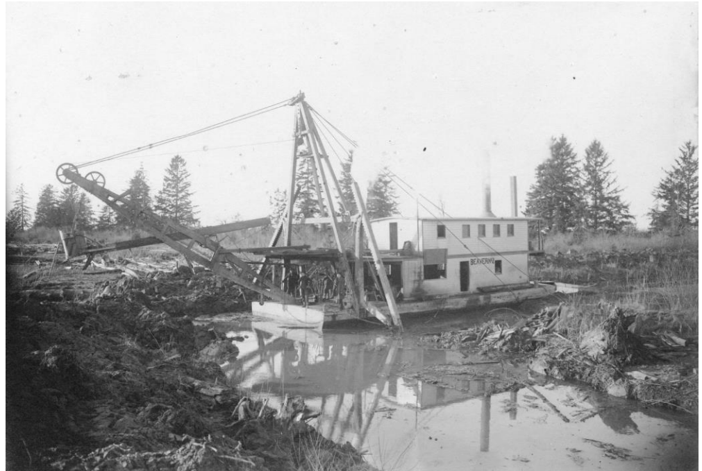
Fig. 7. Dredging Ditches on Lulu Island
