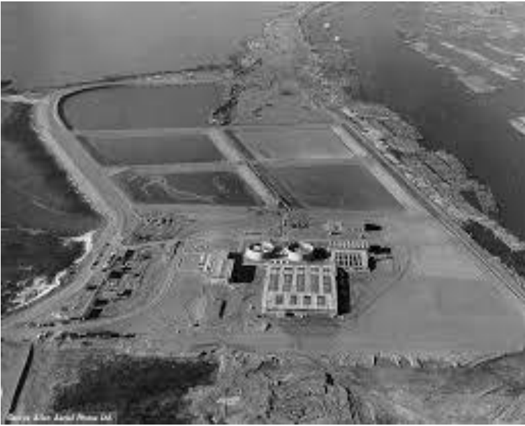
Fig. 87. Iona Island Treatment Plant
