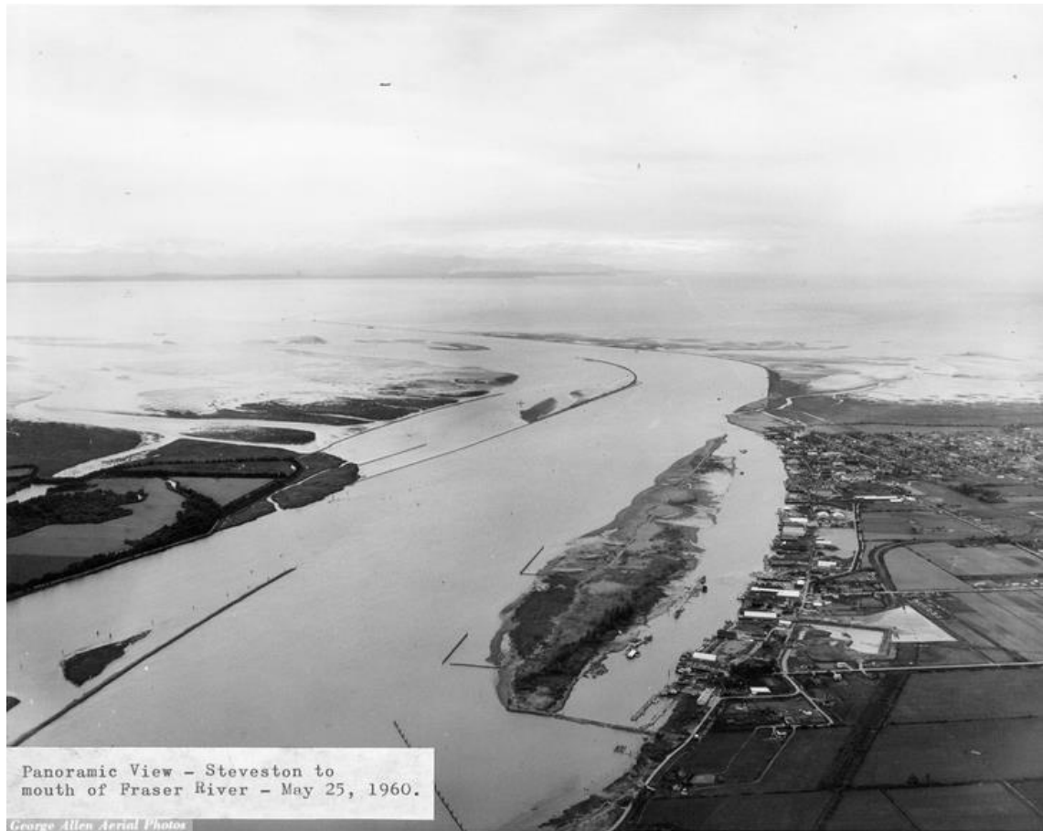
Fig. 102. Aerial of Shady Island and the jetties (1960)
