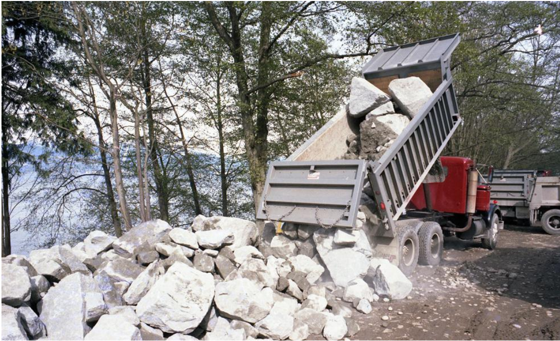
Fig. 75. Armoring the shoreline
