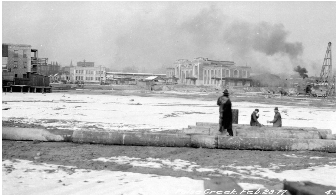
Fig. 48. Workers on CPR rail lot
