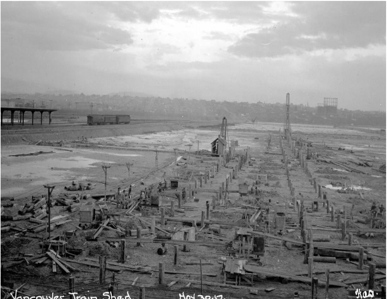
Fig. 47. Construction CPR rail lot
