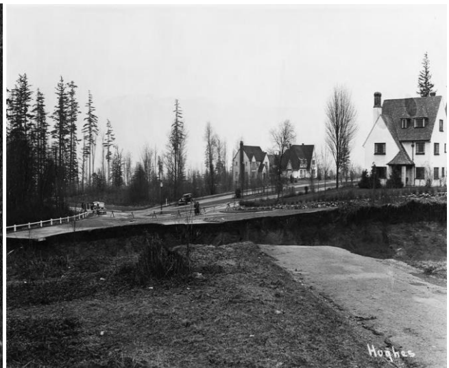
Fig. 68. Graham's Ravine washed out street
