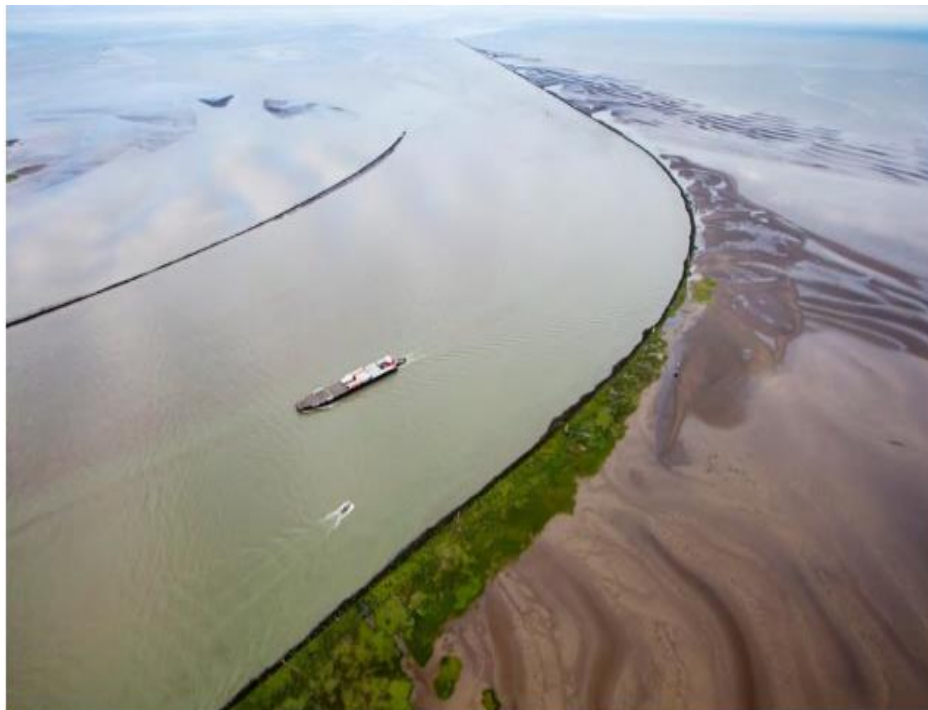
Fig. 107. Marsh along the jetty, current state
