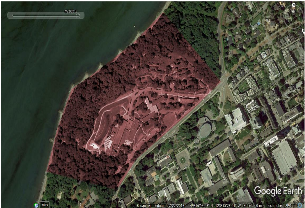
Fig. 78. Area with slope instabilities
