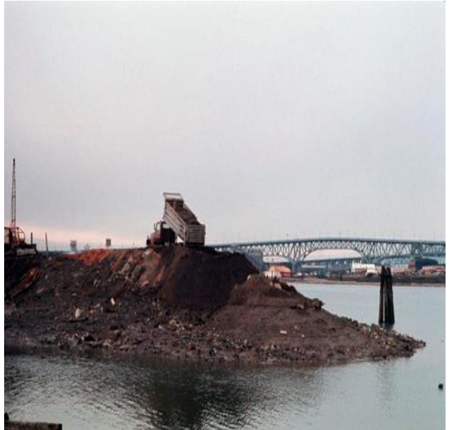
Fig. 56. Construction of the Seawall II
