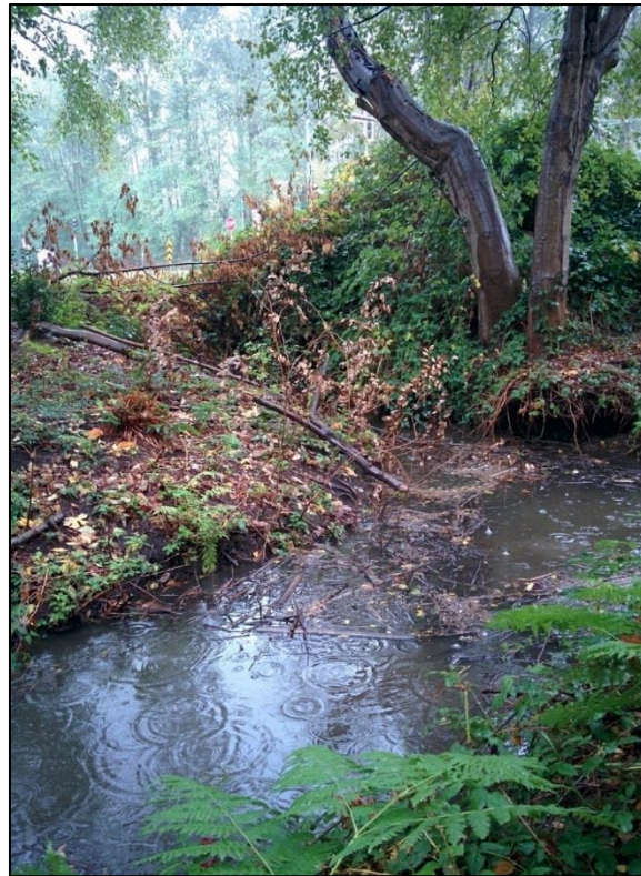
Figure 2-1: Culvert outlet in riparian zone adjacent to Chancellor Blvd.
